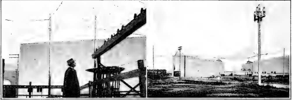
At left, view of aerial screen system and secondary apparatus for collecting charges. At right, public demonstrating screen suspended thirty feet above ground by four poles
